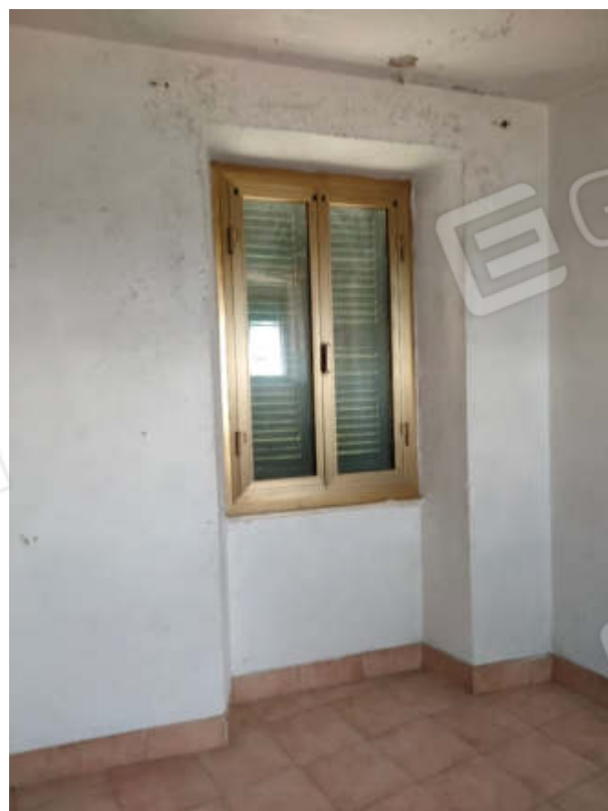
Vista interna rifiniture locale camera in piano primo
