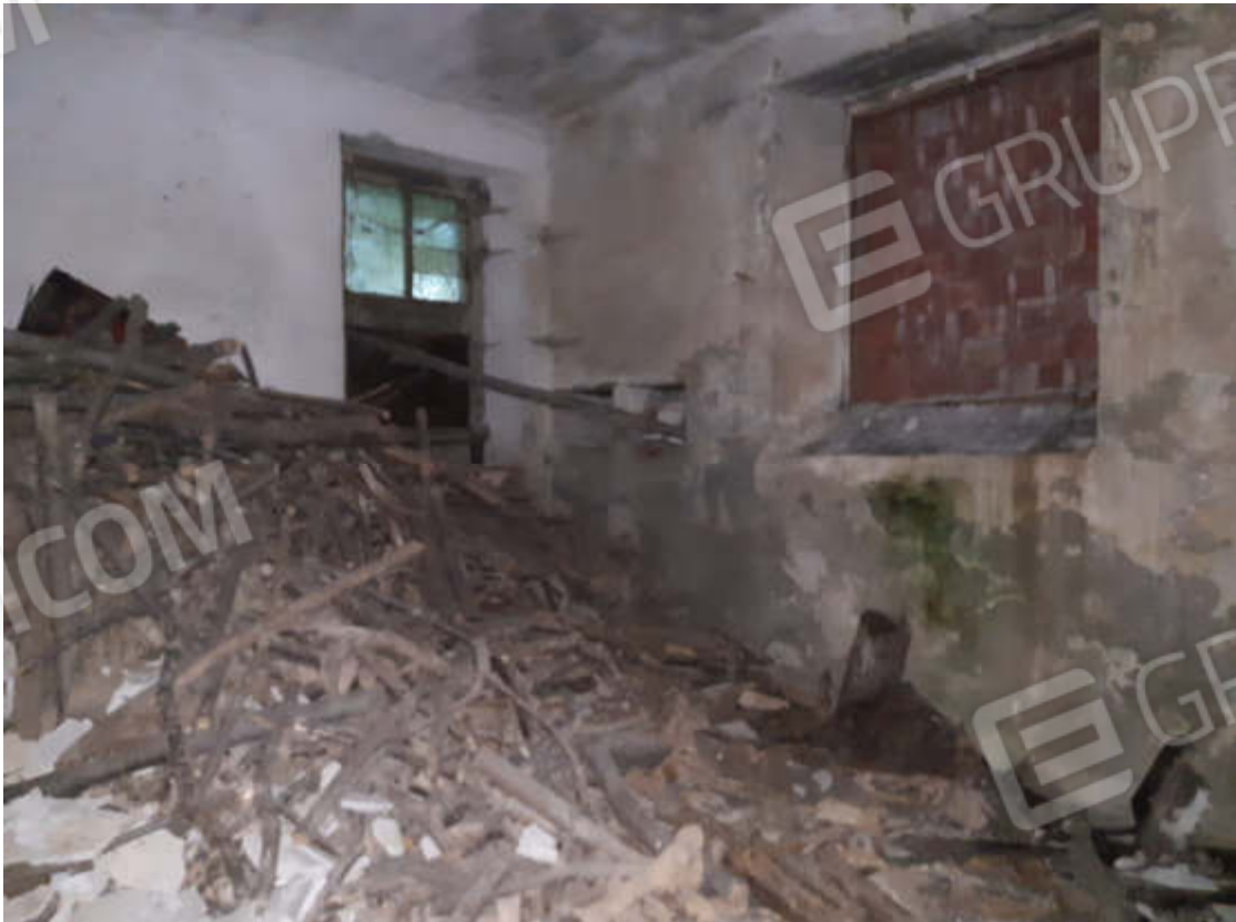
Vista interna locale legnaia in piano terra
