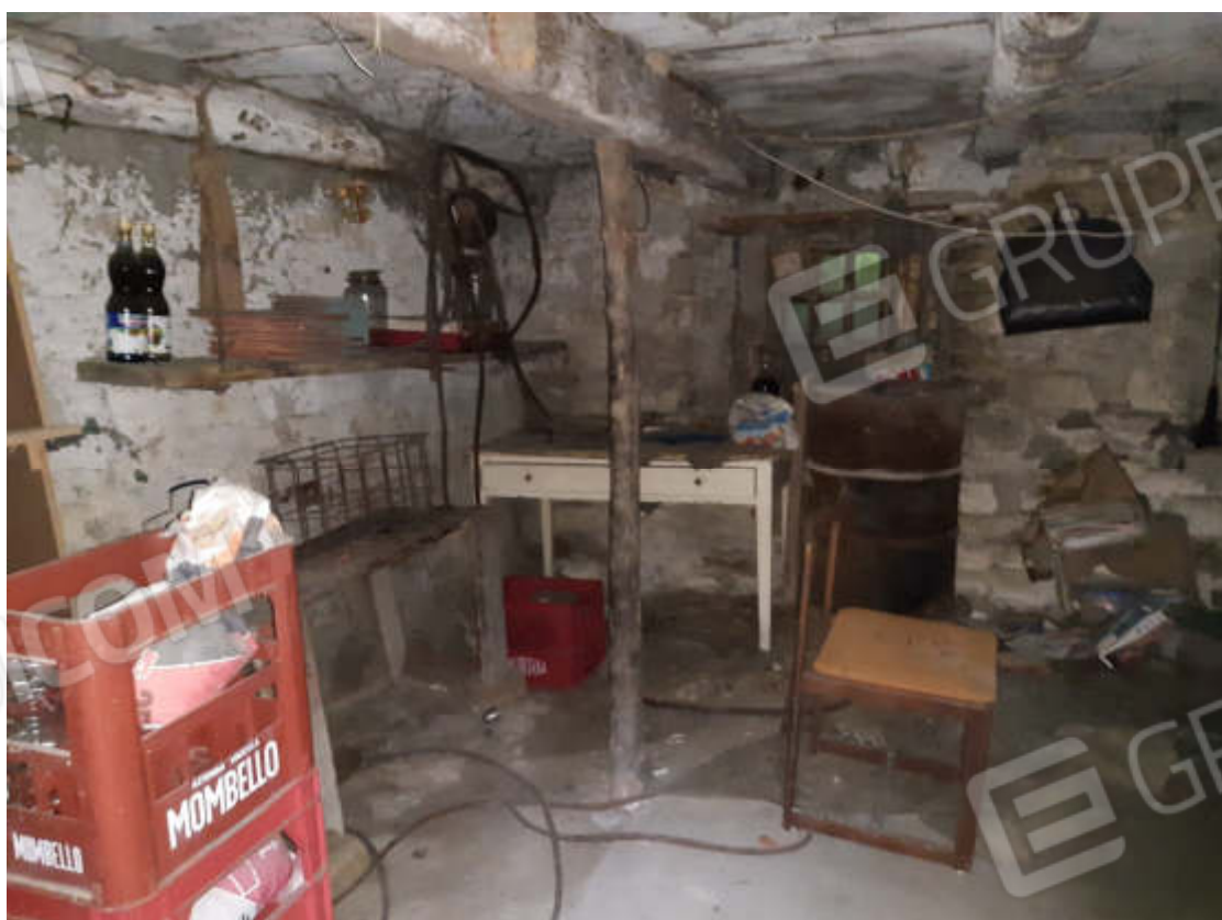
Vista interna locali accessori – cantine – in piano terra
