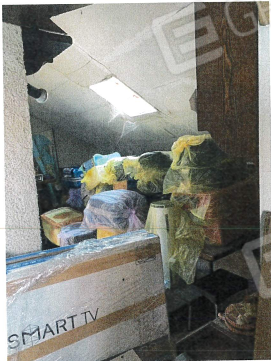
Interno mansarda sub. 6
