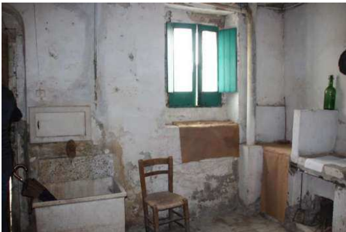
Vista locale piano terra
