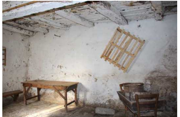
Vista locale piano terra
