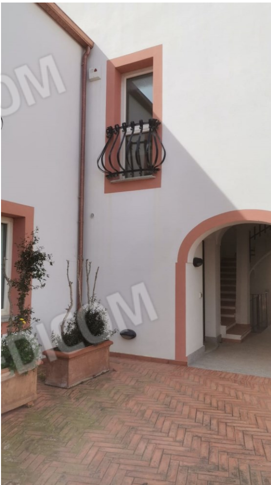
FIGURE 6: A) BALCONE IMMOBILE IN OGGETTO
