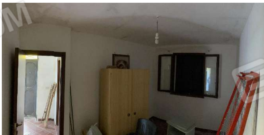
Vano camera piano terra
