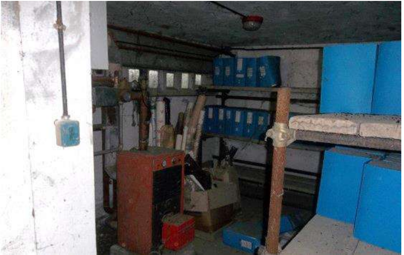
Foto 21 - Piano Seminterrato – C.T. – sub 1
