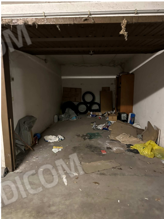
Piano interrato - garage
