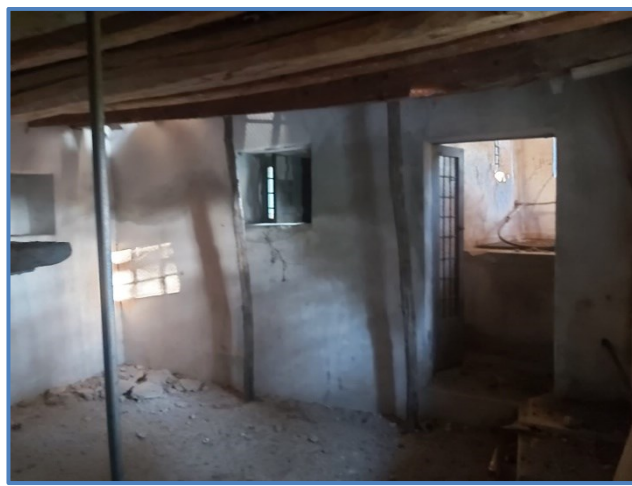
Camera piano terra
