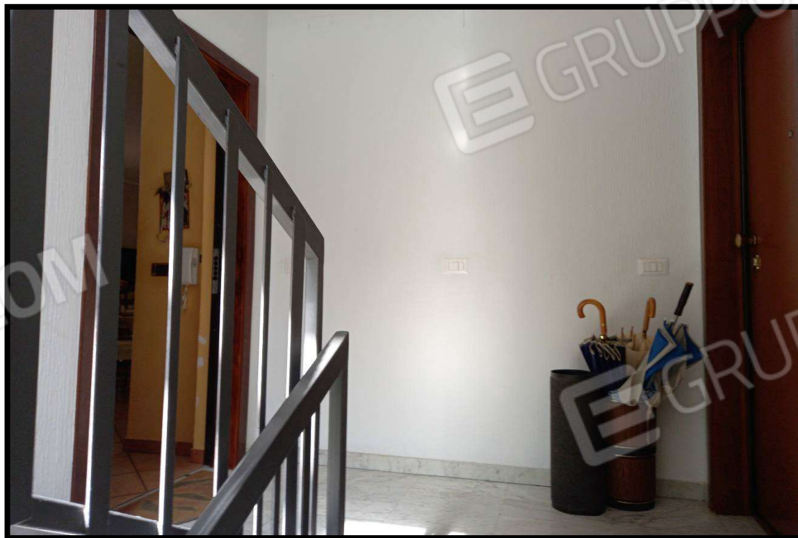
Rampa scale condominiali
