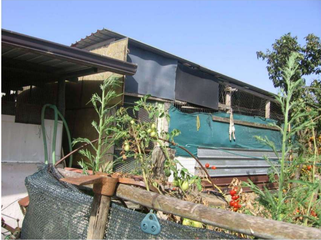
Strutture precarie abusive
