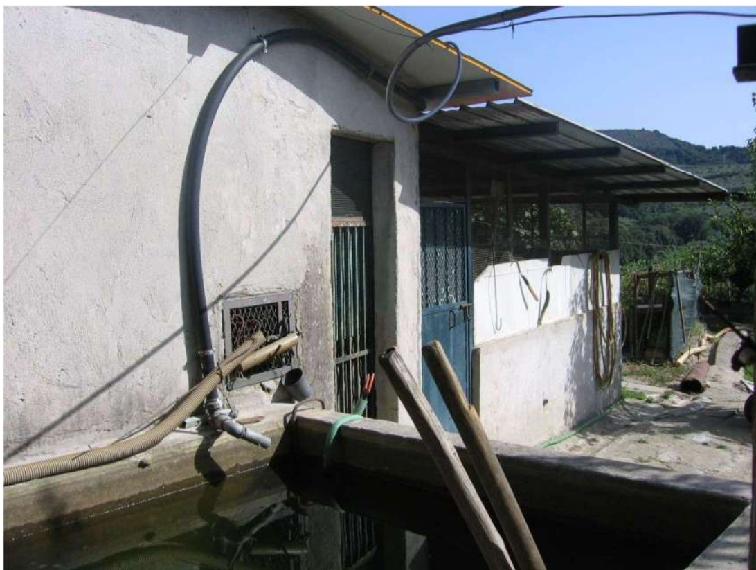
Strutture precarie abusive
