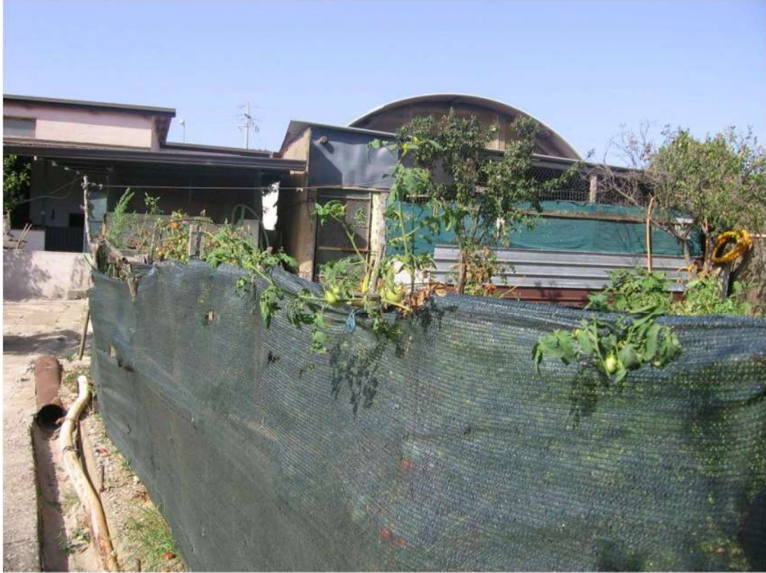
Strutture precarie abusive
