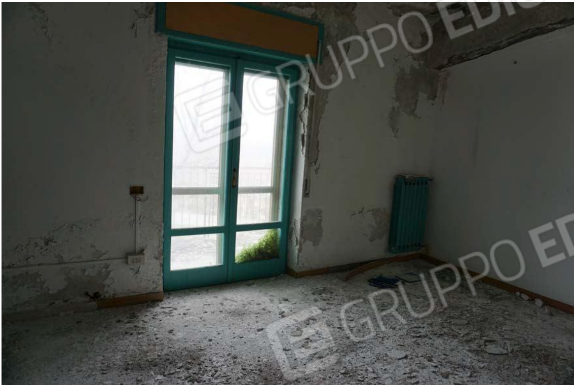
Fig.75 – Vista vano dell’immobile sub.13 (A10)
