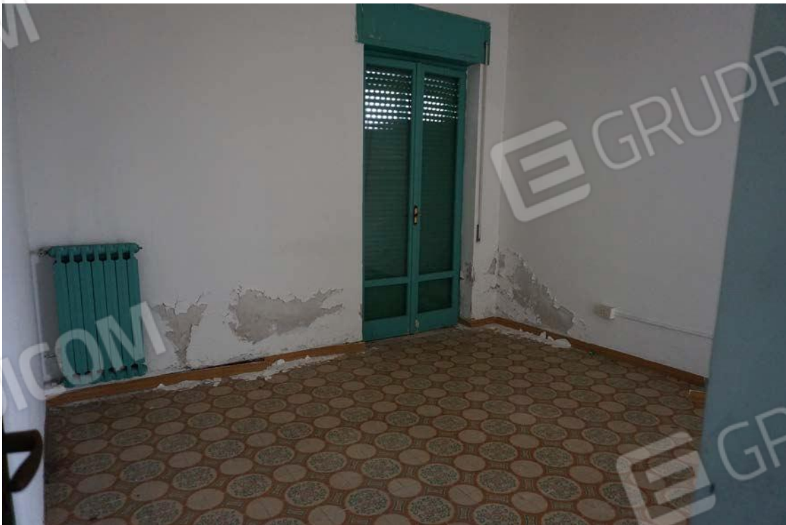
Fig.74 – Vista vano dell’immobile sub.13 (A10)
