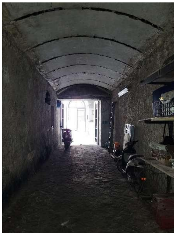
Vista locale box-garage
