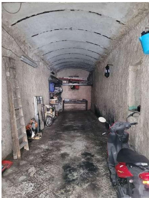
Vista locale box-garage
