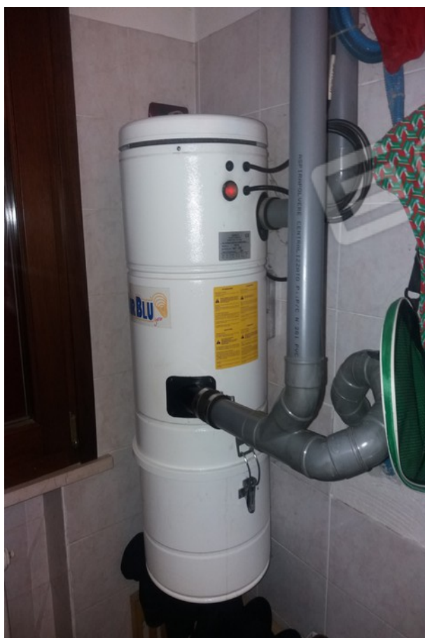
vano C.T. piano seminterrato
