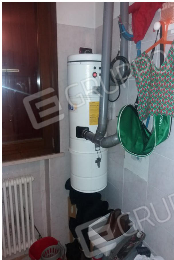
vano C.T. piano seminterrato
