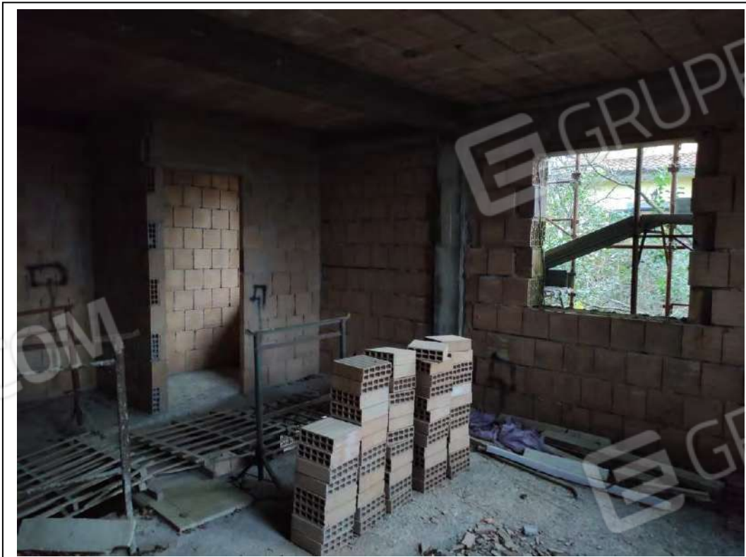
FOTO 14 – Sub. 504 – Piano Terreno
