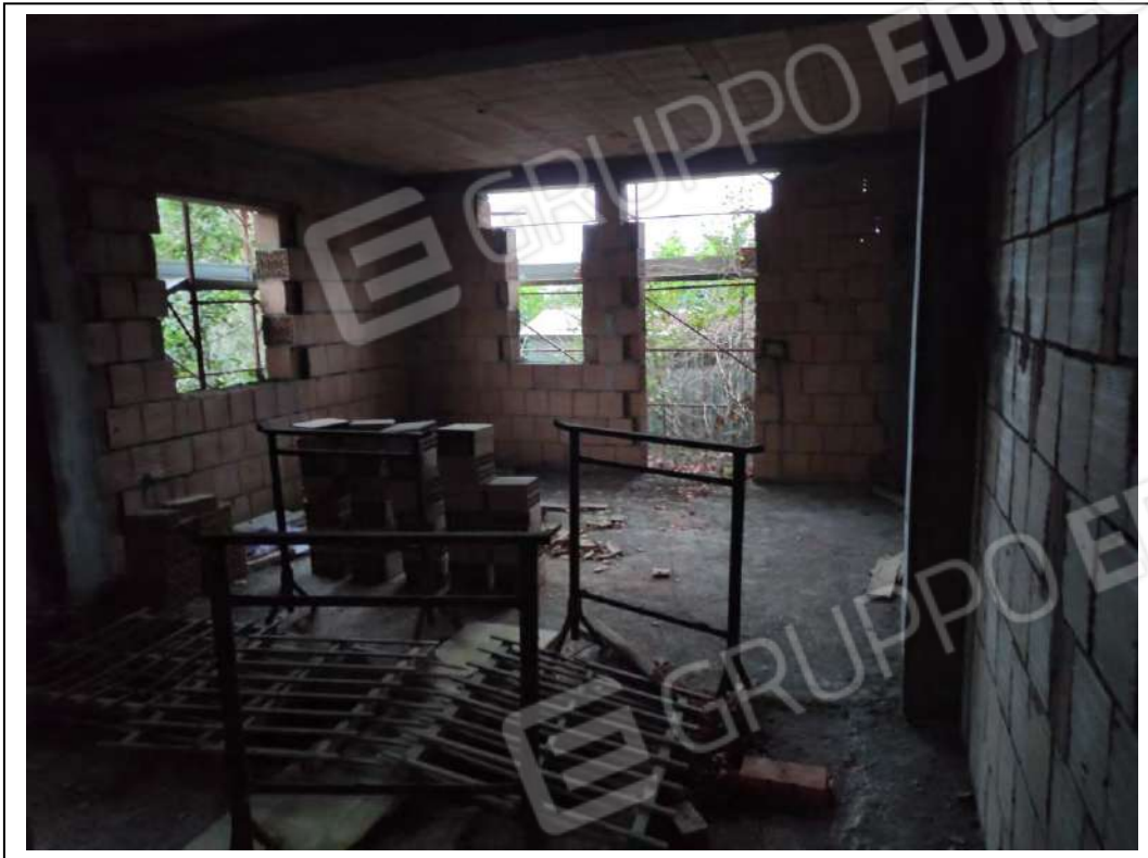
FOTO 13 – Sub. 504 – Piano Terreno
