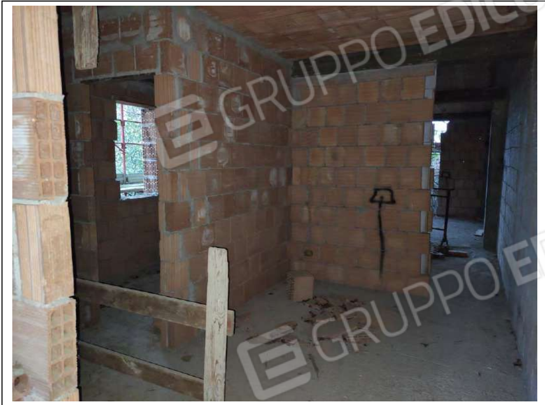
FOTO 11 – Sub. 502 – Piano Terreno
