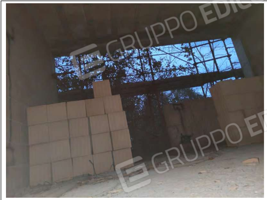
FOTO 15 – Sub. 504 – Piano Terreno
