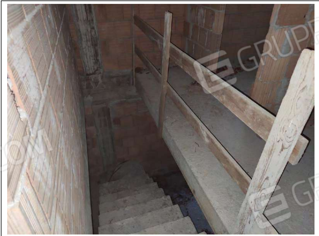
FOTO 12 – Sub. 502 – Piano Terreno
