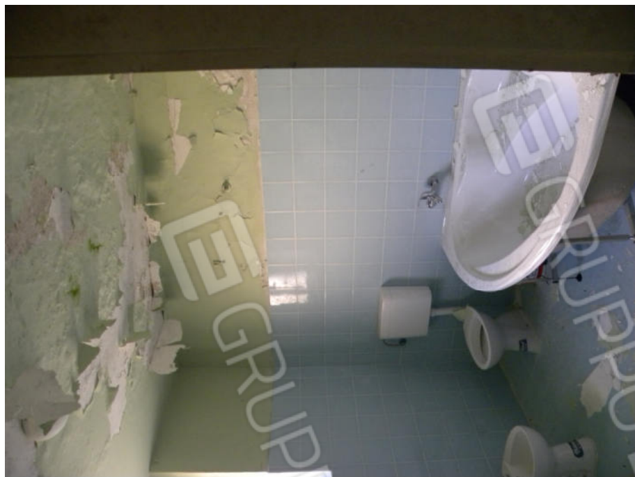
BAGNO PIANO TERRA
