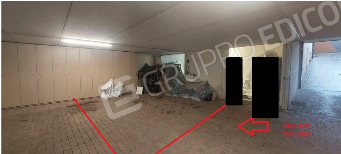
PIANO INTERRATO AREA BOX
