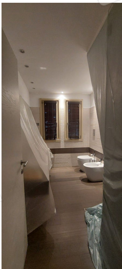
PIANO TERRA BAGNO
