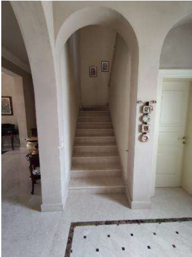
All. 36 – Scala Particella 608 sub. 3
