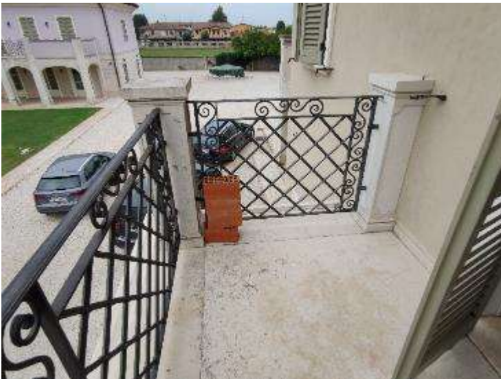
All. 45 – Balcone lato Sud Particella 608 sub. 3
