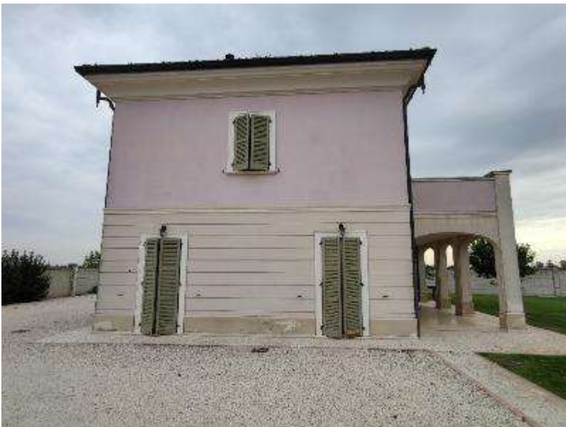
All. 10 – Particella 608 sub. 4 lato Ovest
