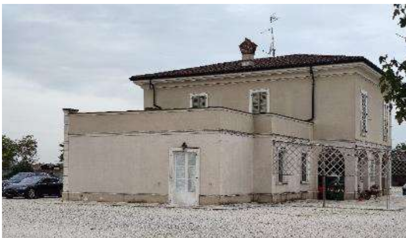
All. 5 – Particella 608 sub. 3 lato Ovest
