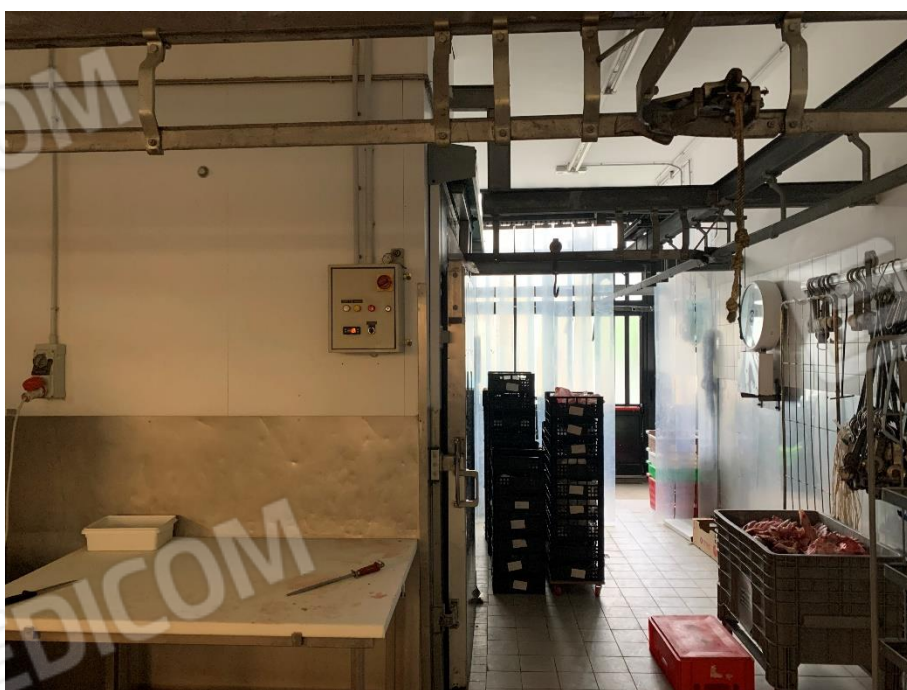
02 locale a piano terreno
