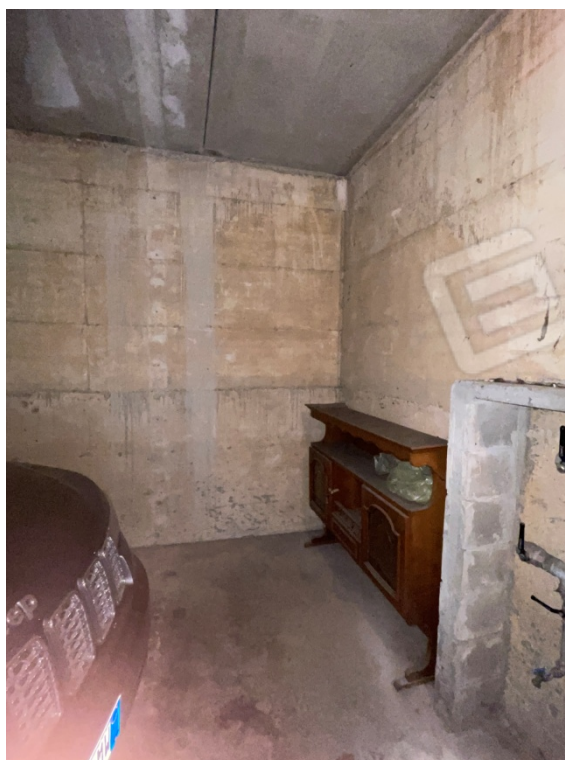
Sub.42 – locale caldaia
