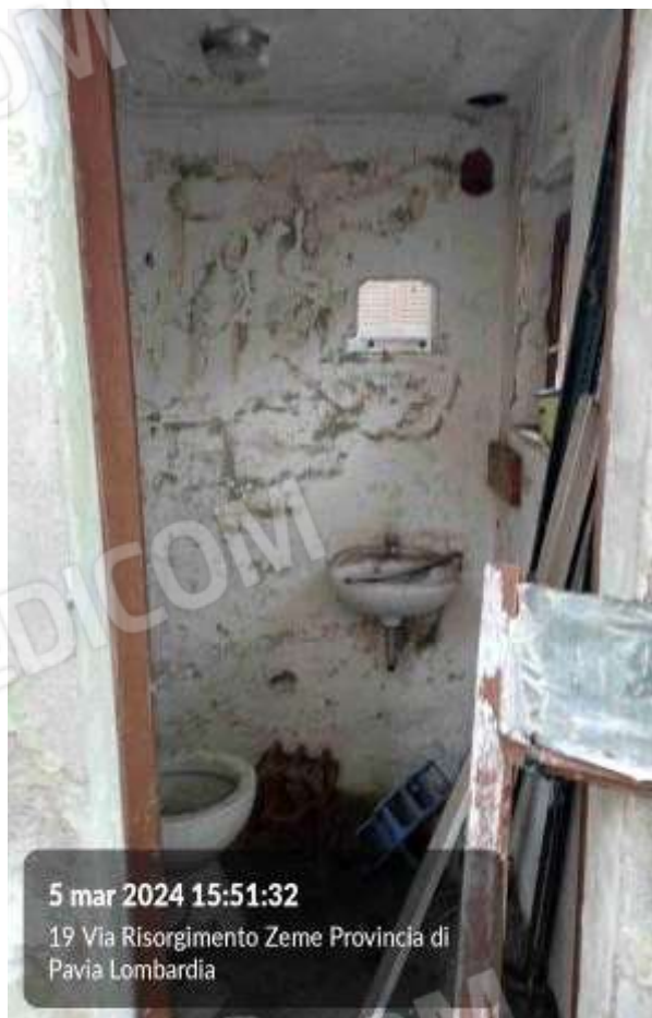
Locale bagno in cortile
